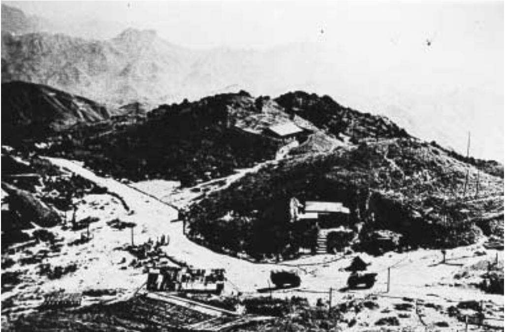
THE JAPANESE RADAR SITE ON TAI MO SHAN – 1942-43
