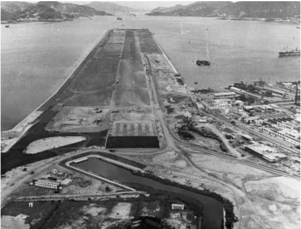
PROGRESS OF THE NEW RUNWAY – MAY 1958
