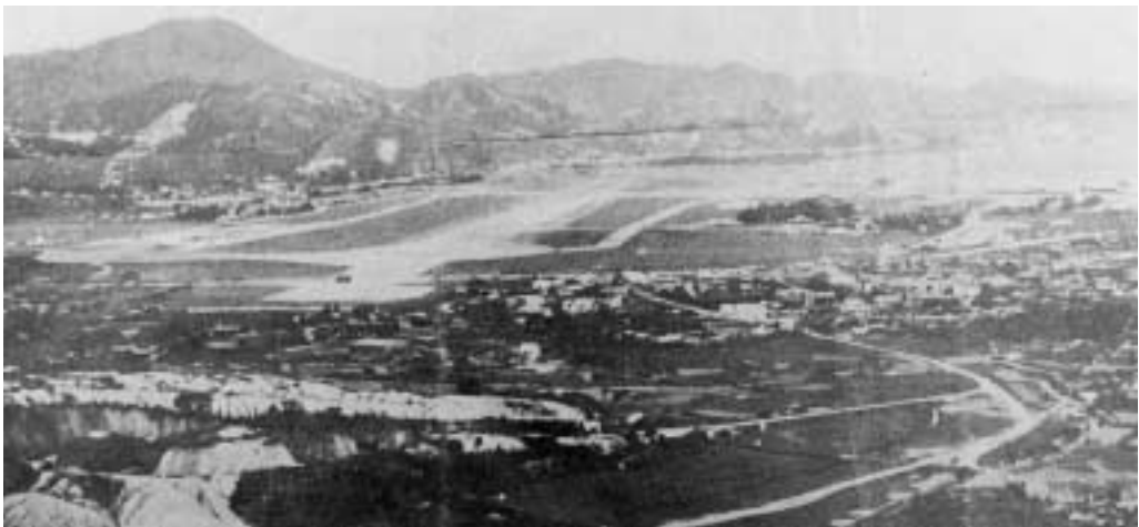
THE EXTENSION TO RUNWAY 13
